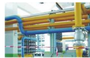
Daishan County Xiushan Seawater Desalination Project
