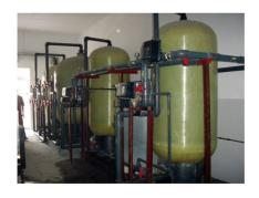
Fleck Dual Tank Continuous Operation Series Water Treatment System Automatic Control Valve
